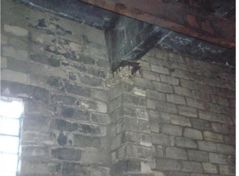
Bricks that supported the roof structure in a very poor state
