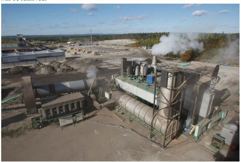
**SAVATERRA Oy - 5. Afterburner** - After cyclone, vaporized contaminants will be burned in an afterburner (oxidiser). Temperature 850-1100 degrees °C destroys the contaminants in to CO<sub>2</sub>.6. Heat exchanger - The flue gas is cooled to 180°C before
