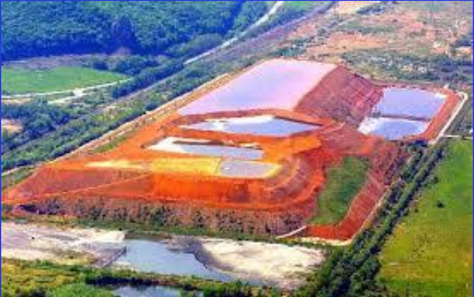
Sludge heap from aluminum production
