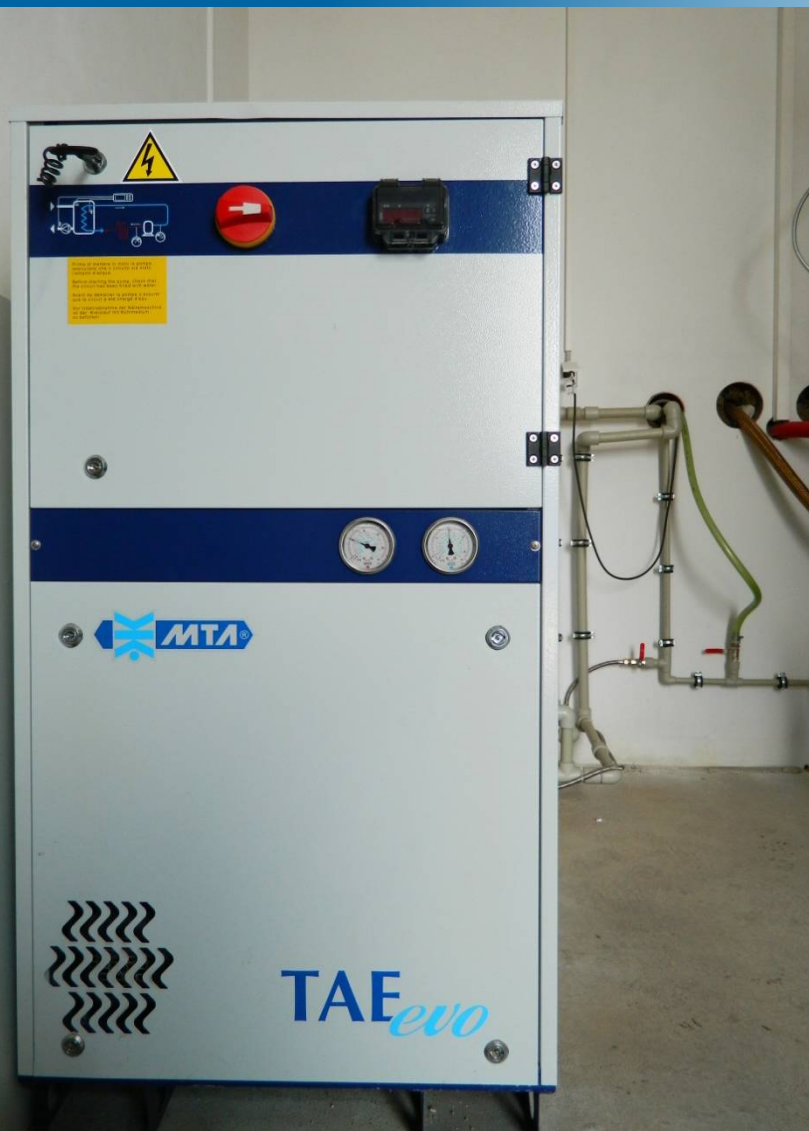
Chiller for cooling water
