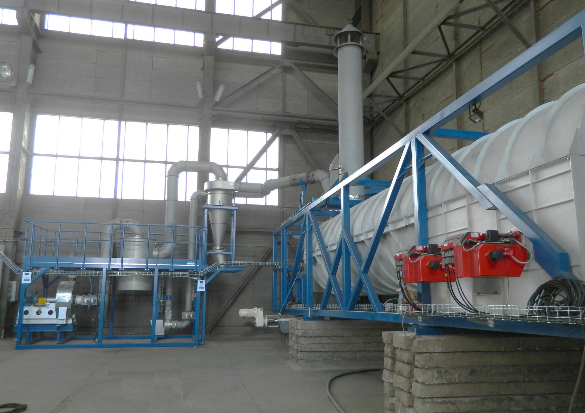
Pilot unit – rotary kiln + off-gas pretreatment
