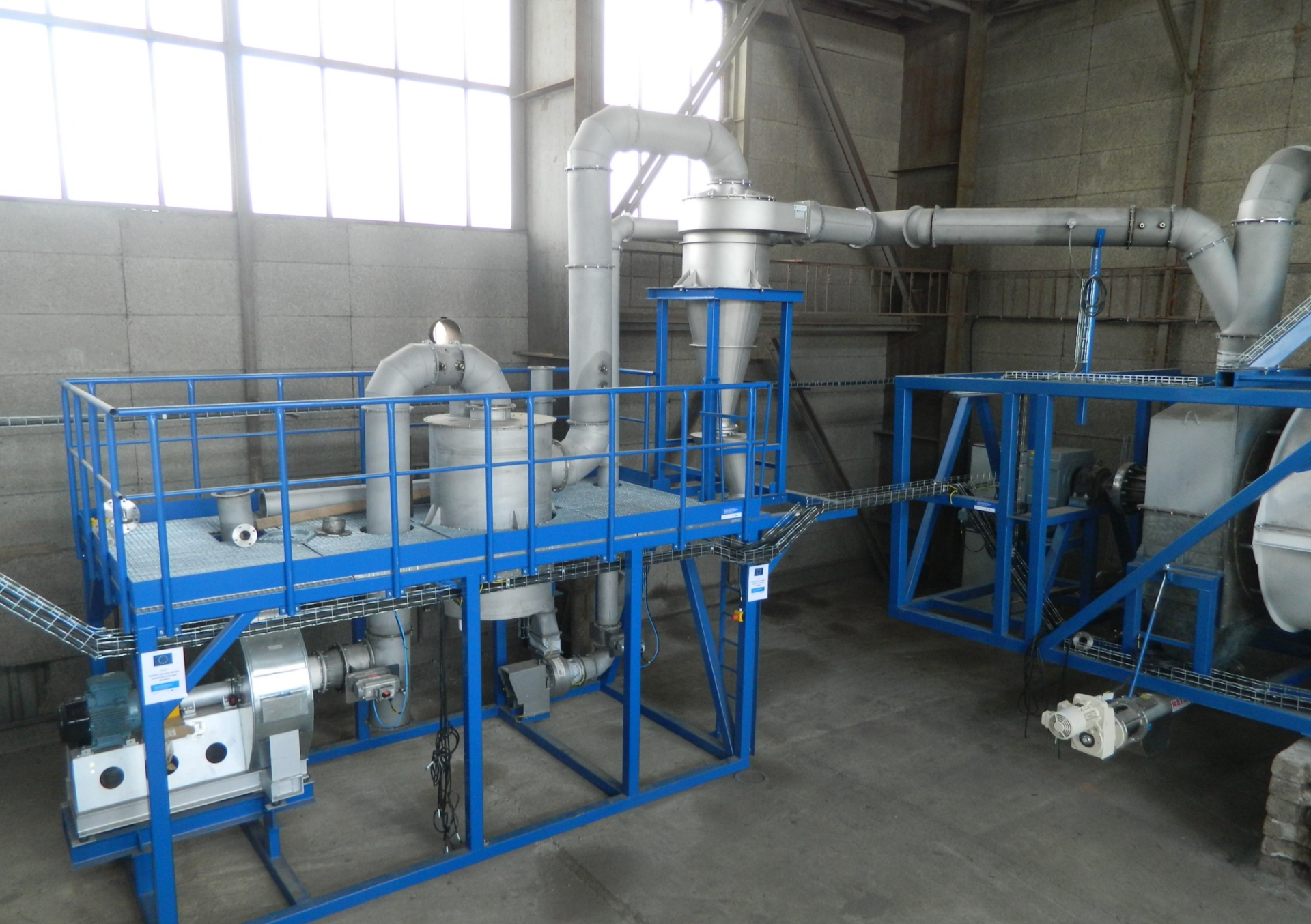
Pilot unit – off-gas pretreatment
