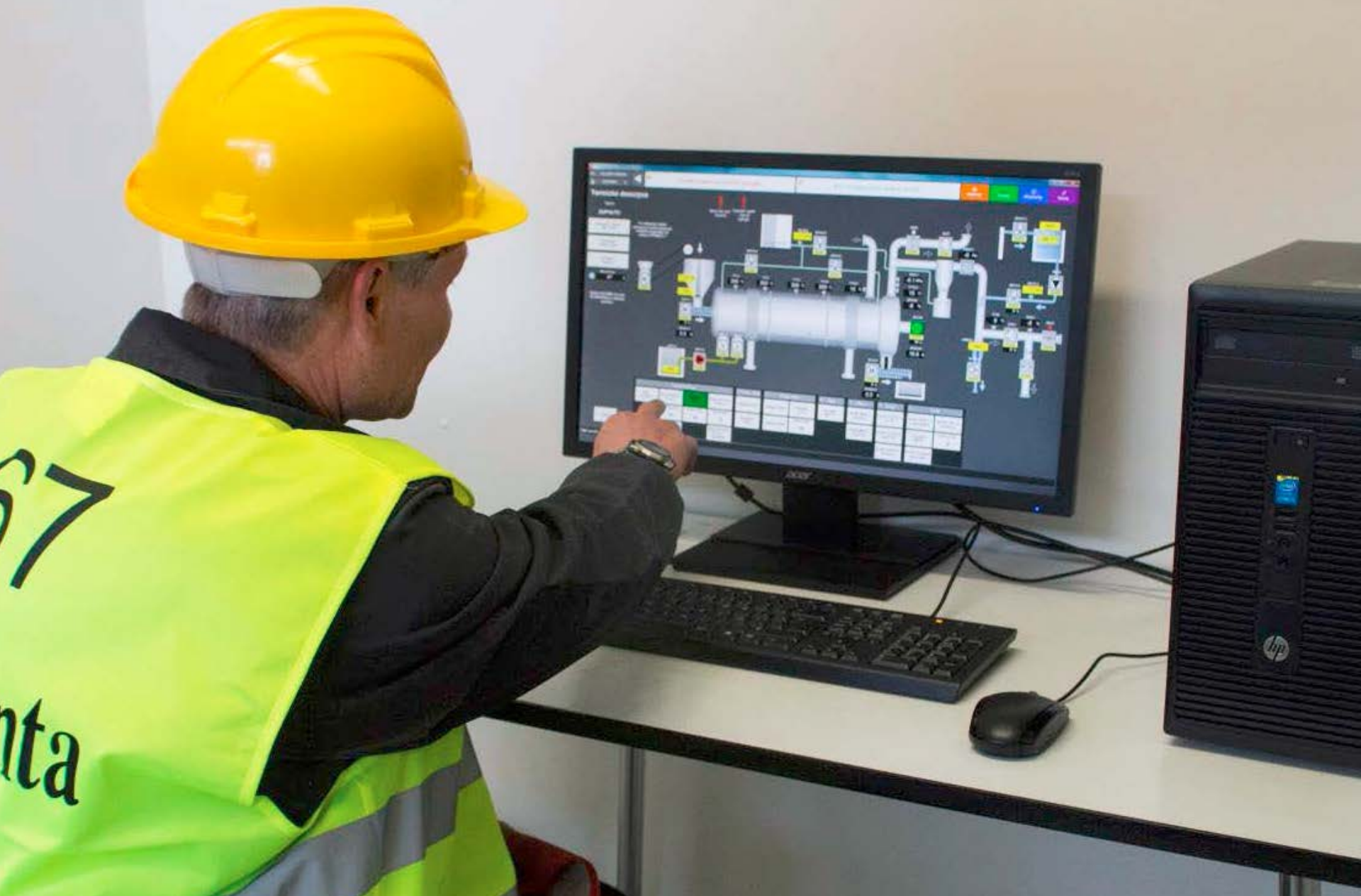
Pilot unit – control cabinet
