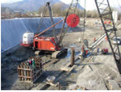
Fig. 1 PRB construction
