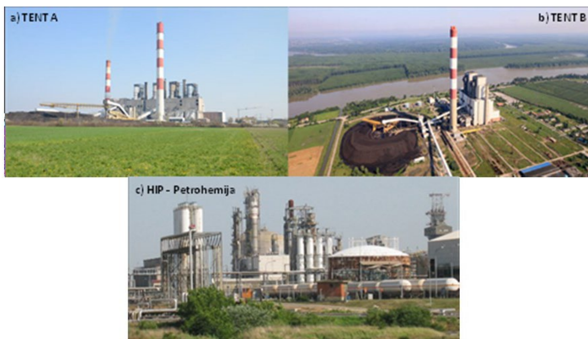
Figure 1. Republic of Serbia, near Belgrade: Nikola Tesla Thermal Power Plants d.o.o. Obrenovac: Tent A (a) and Tent B (b); industrial-petrochemical complex HIP-Petrohemija a.d. Pančevo (c)
