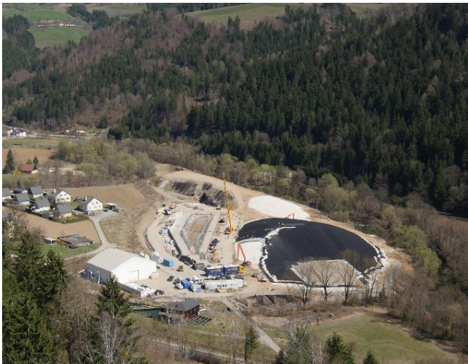
Figure 3. K20 contaminated site (as 28.3.2017) during remediation works
