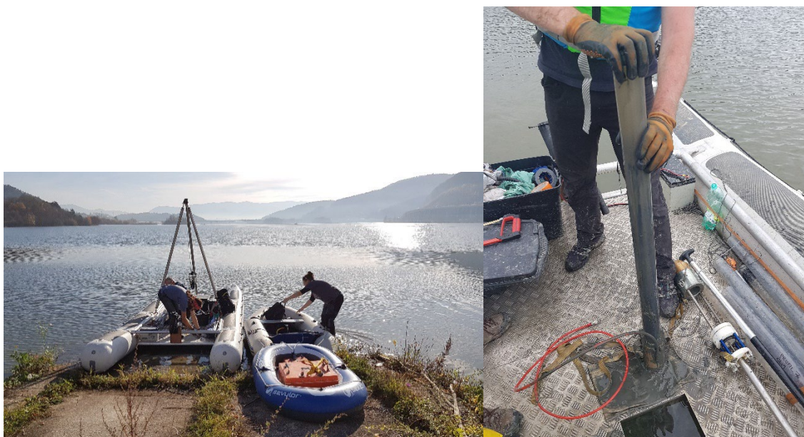
Figure 1. Floating drilling platform and taking the drill core from the bottom of the dam
