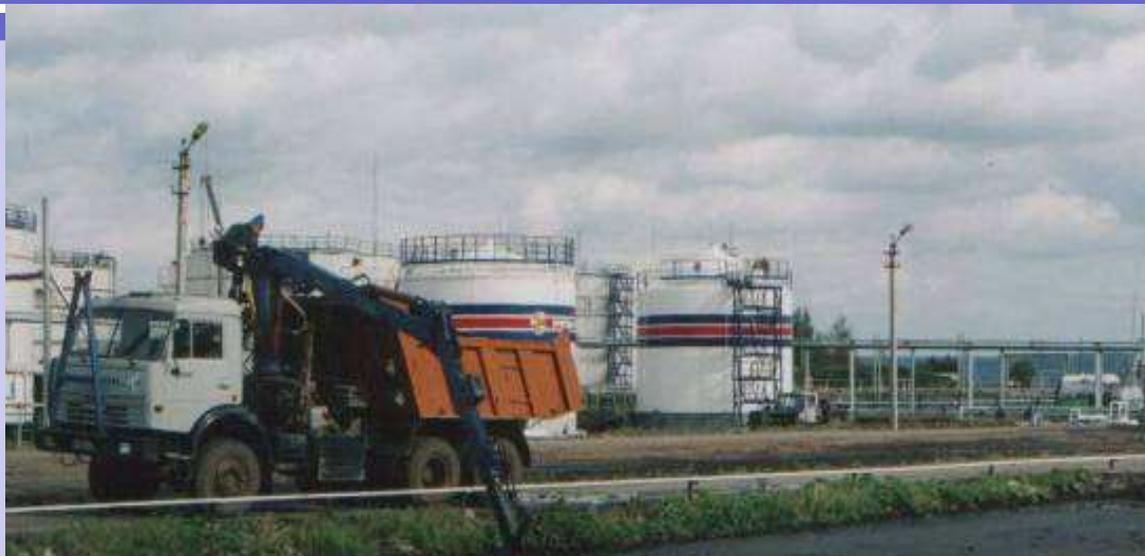
Unloading of OCS from oil waste storage pit using special-purpose machinery
